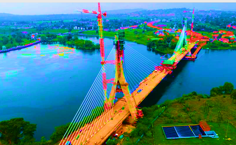
The New Nile Bridge - Jinja
